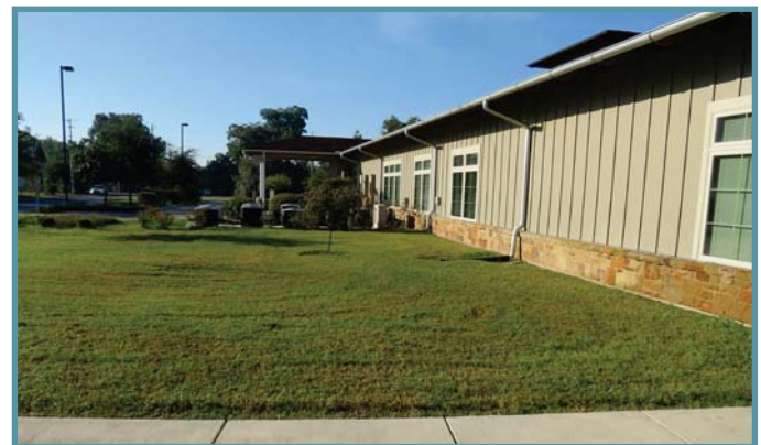
There exist expansion opportunities on the current City Hall property.
