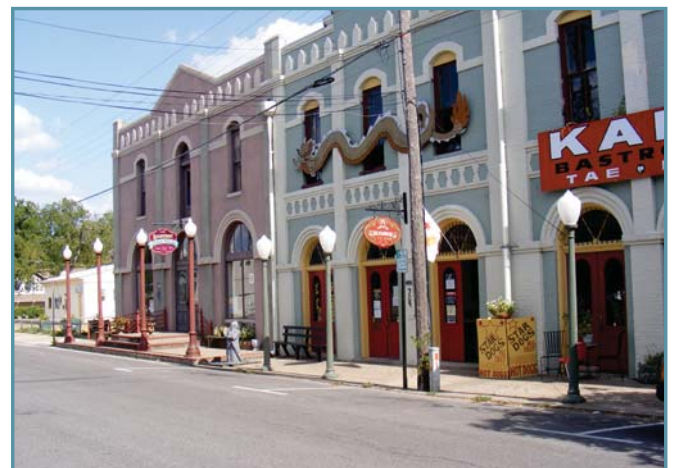
Typical streetscape elements include lighting, plantings, way-finding, and signage.
