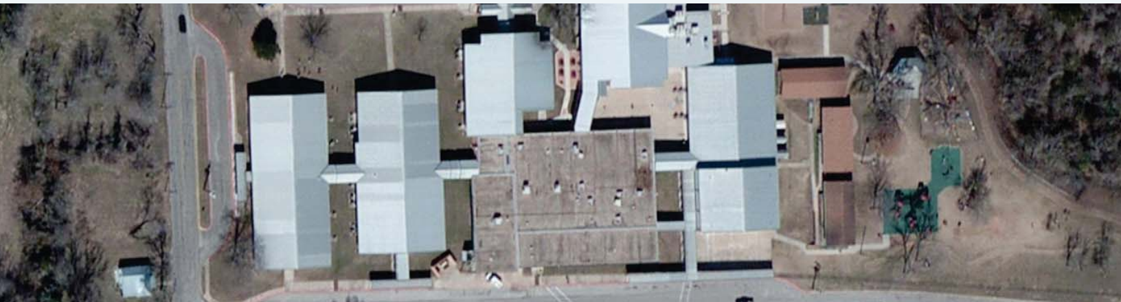
Large-scale civic uses are appropriate in the Public and Institutional character area.
