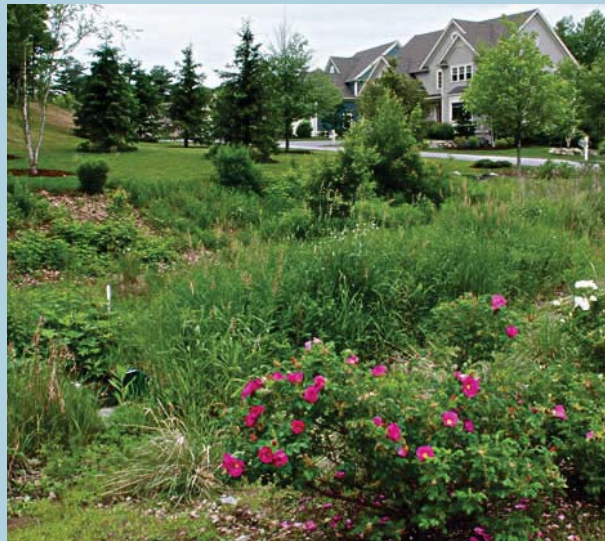
Bio-retention ponds utilize native vegetation to filter pollutants and absorb storm water runoff.
