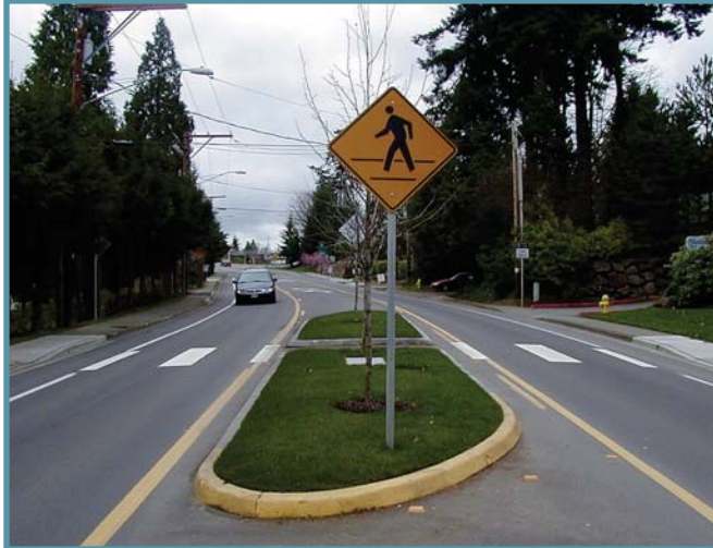
Medians can positively impact both pedestrian and vehicle conditions along roadways. An example median with plantings is shown above.
